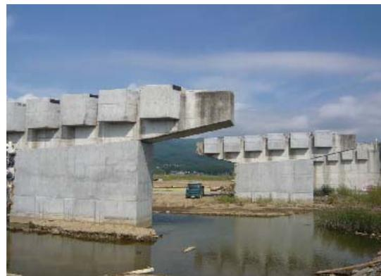
Fig. 5 Damaged Numata-Kosen bridge during Tohoku Tsunami
