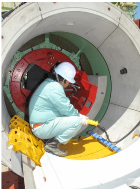
Fig. 6 Secondary lining applied RC segment – assembly
