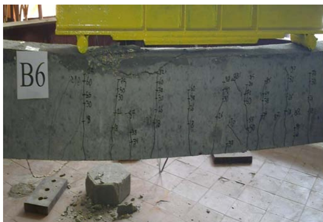
Fig. 7 Typical flexure failure for beam specimens
