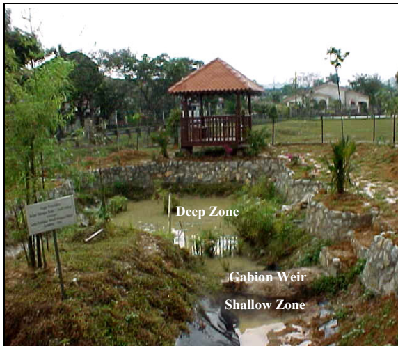
Fig. 1 The constructed mini wet pond located at Sekolah Rendah Kebangsaan Seksyen 2, Puchong, Selangor
