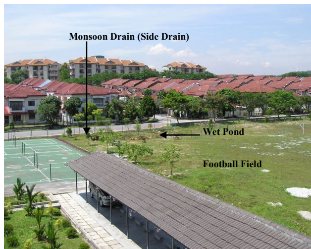
Fig. 2 Catchments of the constructed mini wet pond
