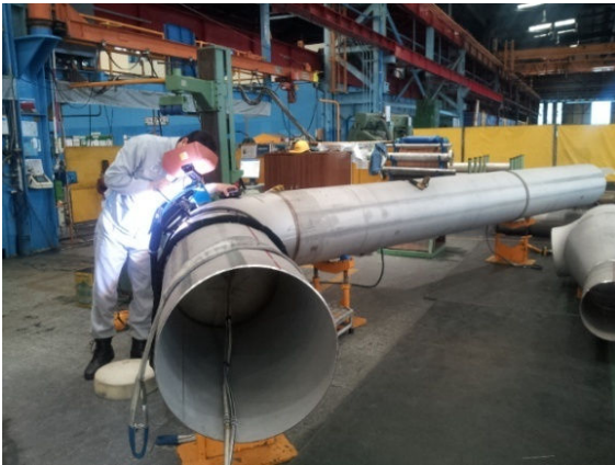
Fig. 8 Stainless steel pipe welding in DSME shipyard
