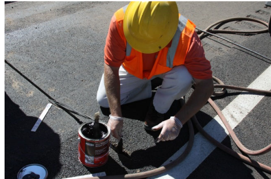
Fig. 6 Installation of temperature probes
