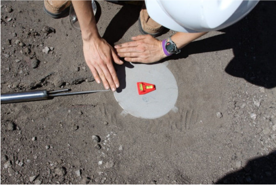
Fig. 4 Installation of earth pressure cell
