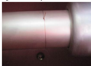
(a) Tip on the high-voltage conductive pole
