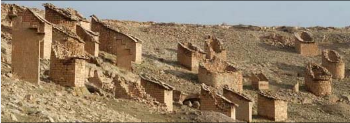
Fig. 12 The dovecotes with chimneys at Nevşehir region [8]
