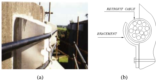
Fig. 3 (a) Retrofit post-tensioned cables, (b) Detail of post-tensioning cable saddles.
