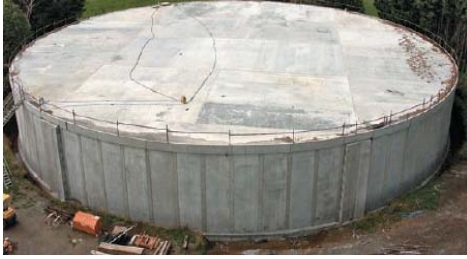
Fig. 2 Completed 20000 m 3 , pre-cast concrete reservoir.
