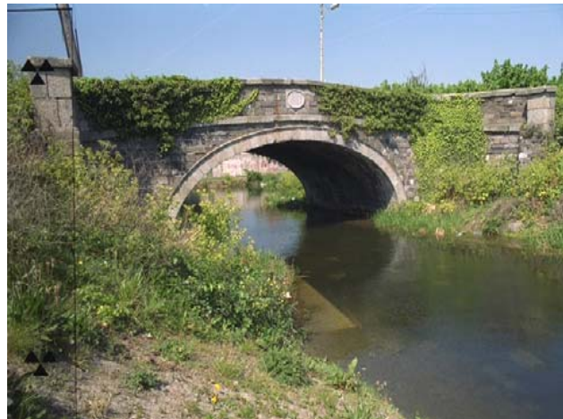
Fig. 1 Griffith Bridge – Dublin
