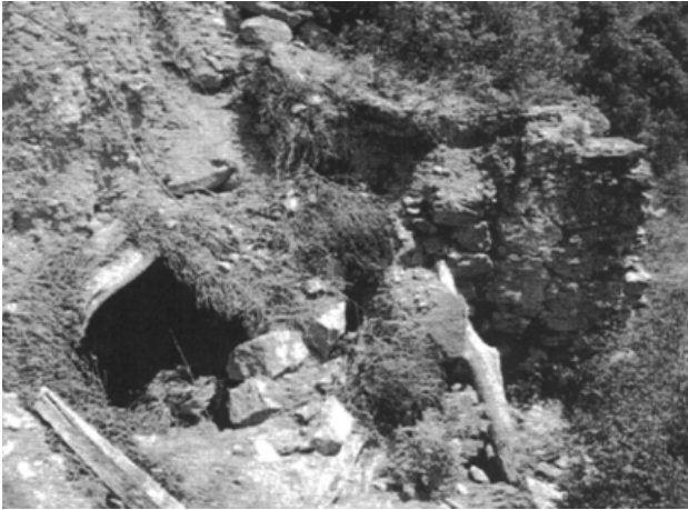
Fig. 6 Lime Kiln 2 as seen from the access path
