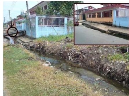
Fig. 1 Housing area on low-lying peat soil ground, Jalan Lai Chee, Sibü.
