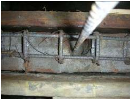
Fig. 5 Reinforcement Details @ junction
