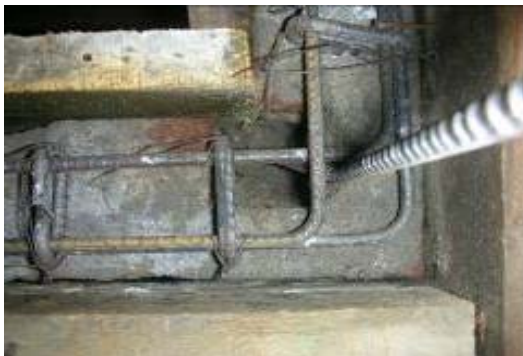
Fig. 6 Reinforcement Details @ corners
