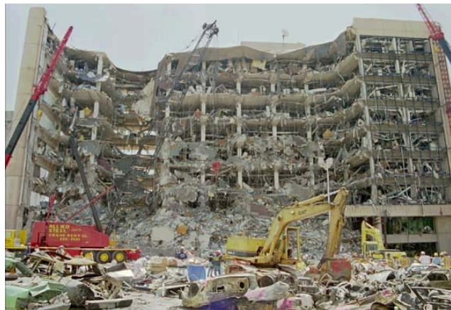
Fig. 2 Alfred P. Murrah Federal building after the 1993 bomb attack [2]
