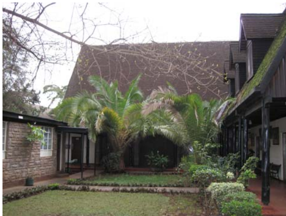
Fig. 11. Main Building at the Nairobi Zoo, Kenya. The use of 'cavaco' for the roofing. A technology extensively used by the Ribeirinhos and the indigenous people in the Amazon region.
