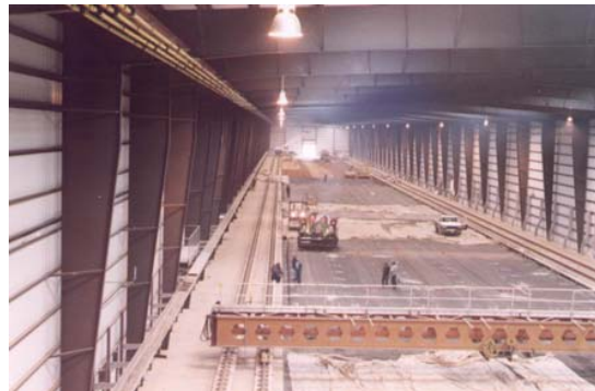
Fig. 1 Inside view of NAPTF during construction of test pavements (Photo Courtesy: NAPTF)
