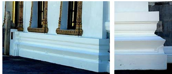
Fig. 5 The basement "Lion Basement" of Amarindra-vinijchai-mahaisuraya Bhiman throne hall
