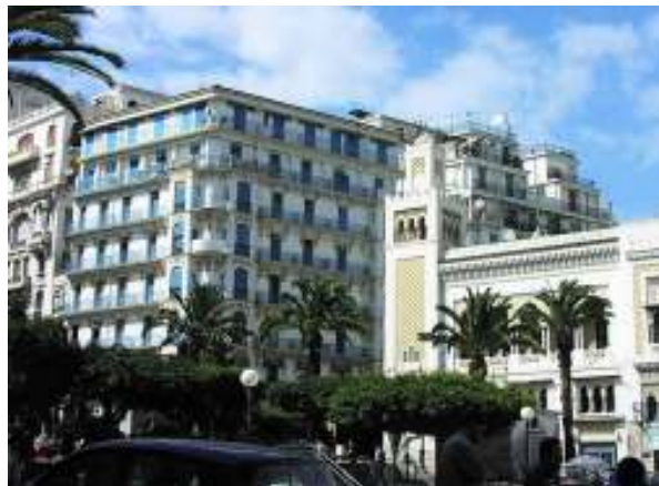
Fig. 3 Town of Algiers – masonry buildings
