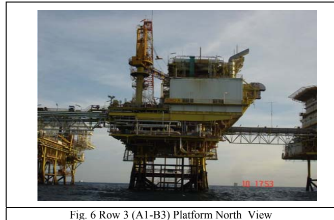
Fig. 6 Row 3 (A1-B3) Platform North View
