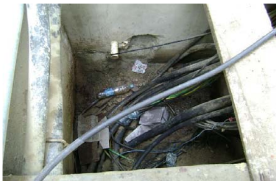
Fig. 14 Electric cable trench was found uncovered
