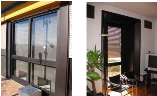
Fig. 1 Outside and inside view of solar wall
