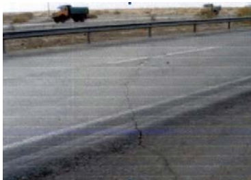
Fig. 5. Fissuring in Yazd-Maybod main road
