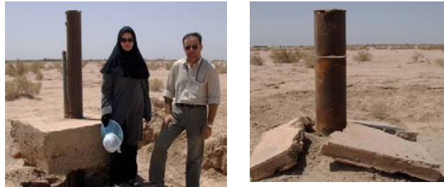
Fig. 4. The growth of water wells casing due to land subsidence
