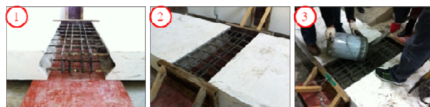
(a) Precast members (b) Setup the mold (c) Placing concrete
