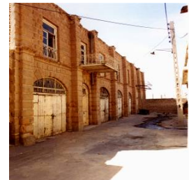
Fig. 3 Multi storey buildings
