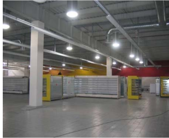
Fig. 3 Storeroom illuminated by light pipes
