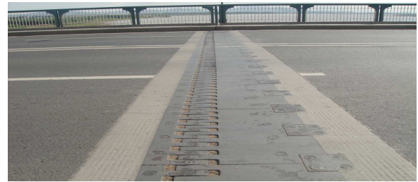
Fig. 4 (a) Joint fill with dust
