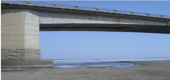
Fig. 1 (b) T-shape cantilever structure
