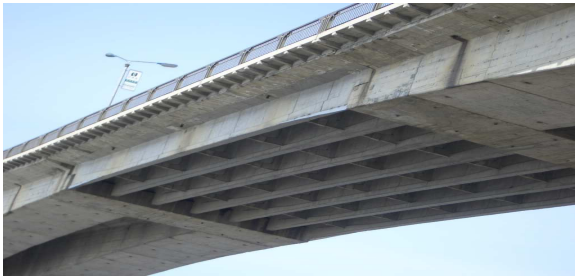
Fig. 1 (c) Hanging beams
