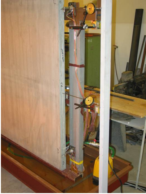
Fig. 5 Sprinkling glass-fiber-concrete façade panel: view to indicators of deformations on the side of specimen
