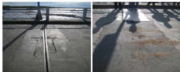
Fig. 11 Serious damaged bridge deck expansion joint
