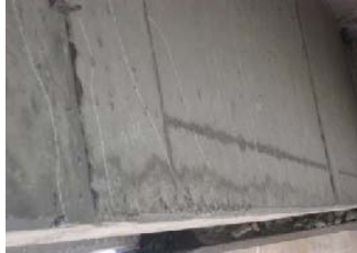
Fig. 9 (b) T beam cross-cracks in the region
