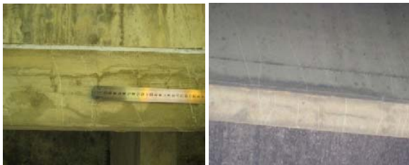
Fig. 9 (c) T beam cross-cracks in the region
