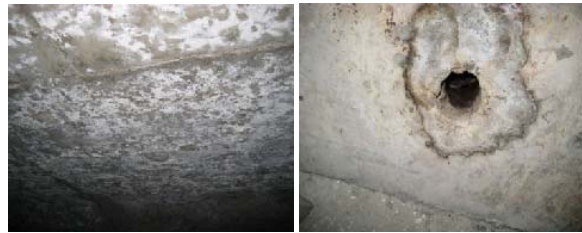
Fig. 9 (a) the internal box water drainage damage
