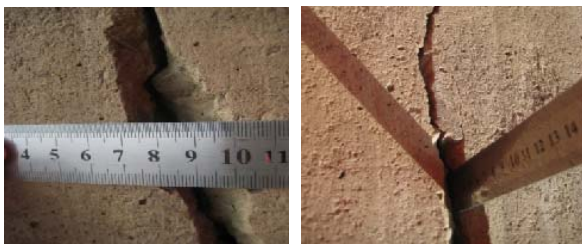
Fig. 5 5 Pier # 5 crack depth
