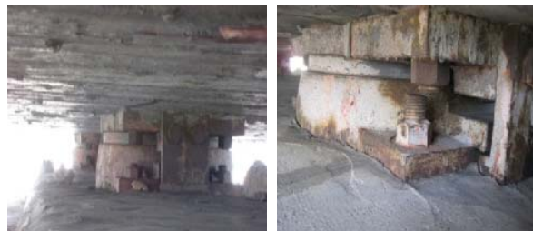
Fig. 8 Bearing steel plate
