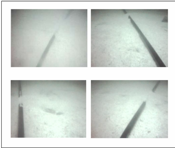
Fig.6 Typical examples of occluded pipeline
