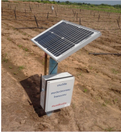
Fig. 10 SSN base station (Coordinator) installation in SUT farm
