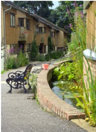
Fig. 6 Planted 'rill' at Springhill Housing, Stroud, UK (c/o Robert Bray)
