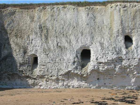
Fig. 3 Cavities of typical piping / sapping erosion [6]
