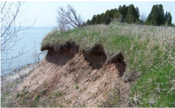
Fig. 2 Collapse of layer undercut by piping / sapping [6]
